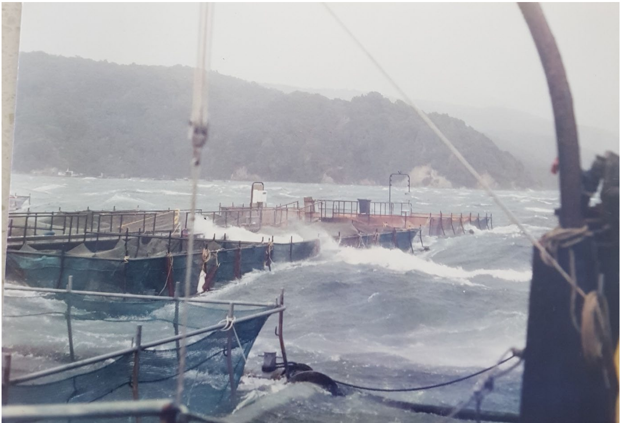
The farms at Big Glory Bay had to be built to withstand some rough conditions
